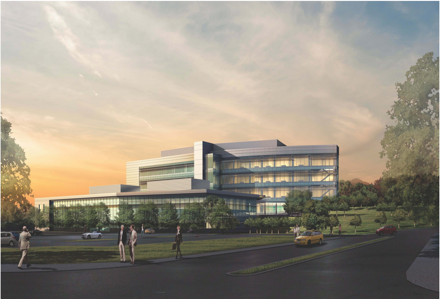
Rendered image of East County Hall of Justice in Dublin, CA—scheduled for completion in 2017
