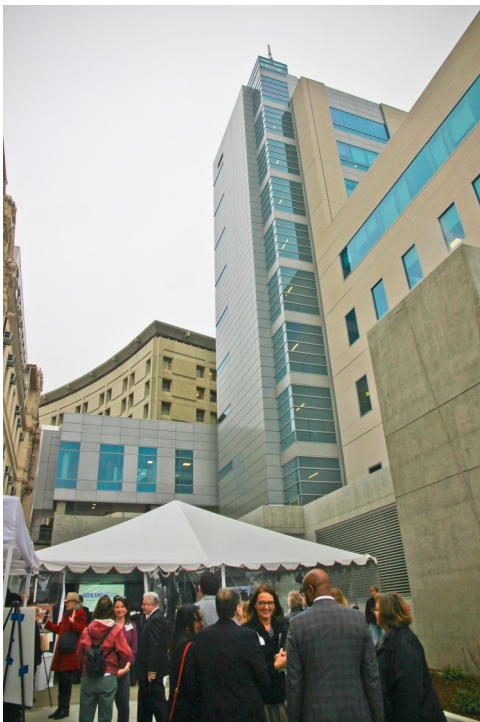
The Highland Hospital Acute Tower Replacement Project. Alameda County's largest capital project, scheduled for completion in 2017
